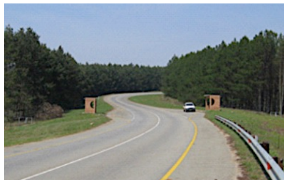
Figure 4 More sustainable infrastructure in Swaziland
