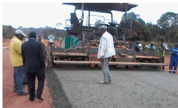
Figure 19 Construction of rural roads in Cameroon
