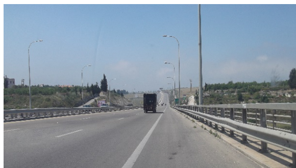
Figure 18 Southern Coastal Highway in Lebanon
